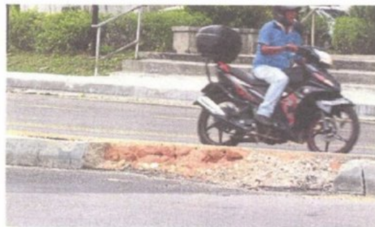
The one-way loop has parts with broken road medians. The project is still ongoing but the quality of the construction is questionable. — filepic
